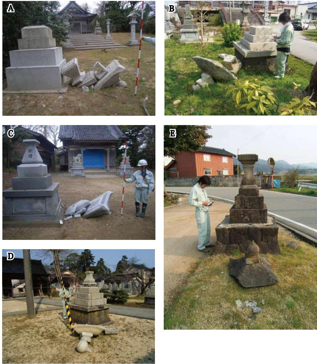
FIGURE 20. Field occurrences of overturned Joyato-type stone lanterns. A–B, Overturning of parts above a pedestal. C–D, Overturning of parts above a column. E, Overturning of parts above a middle platform.
