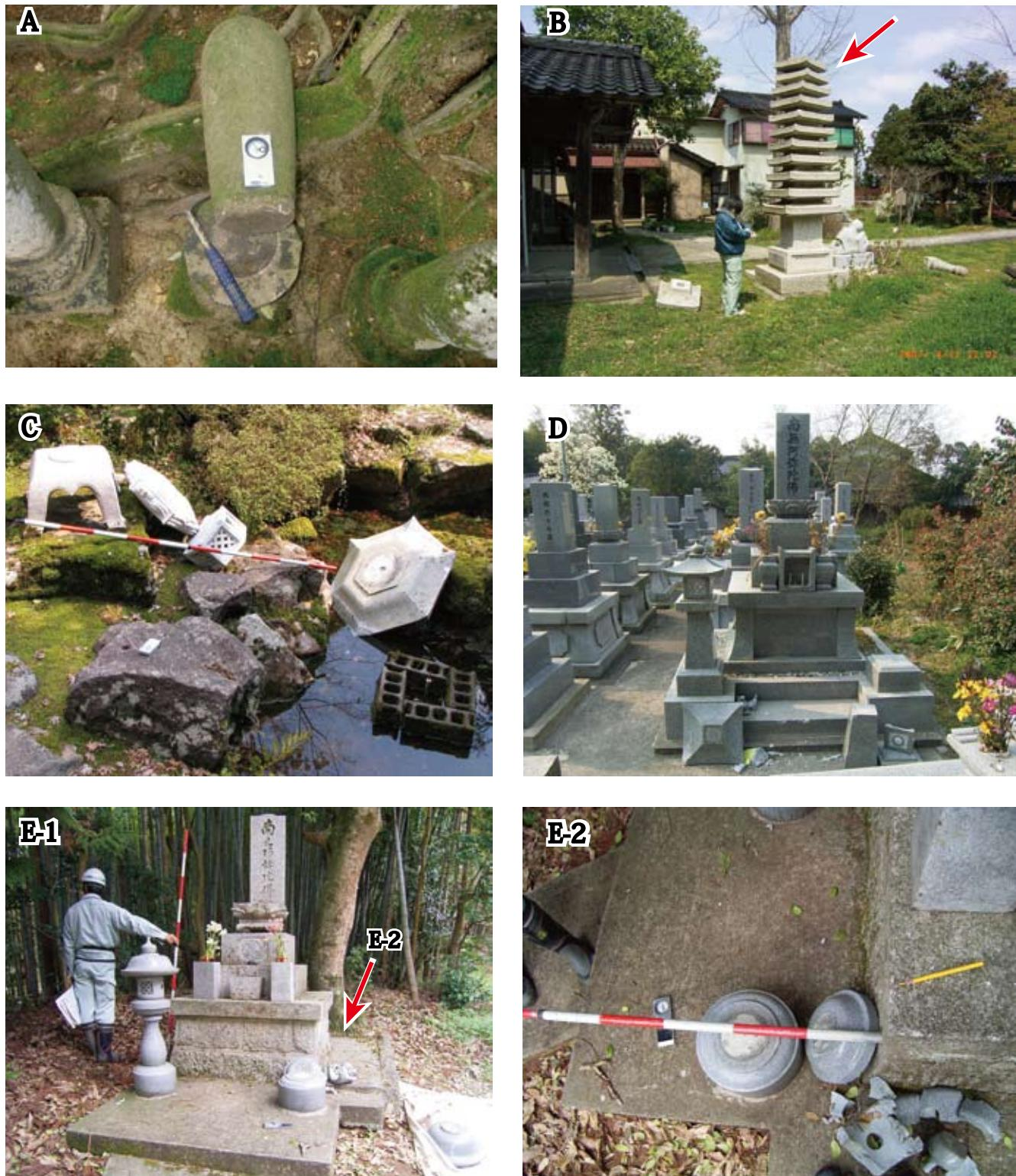
FIGURE 16. Field occurrences of various types of gravestones and stone lanterns. A, Overturning of Muohoto-type gravestone. B, Overturning of pagoda (thirteen-stories). Red arrow shows some rotated roofs. C, Overturning of Yukimi-type stone lantern. D, Overturning of Kakubozan stone lantern. E, Overturning of Marubozan stone lantern.
