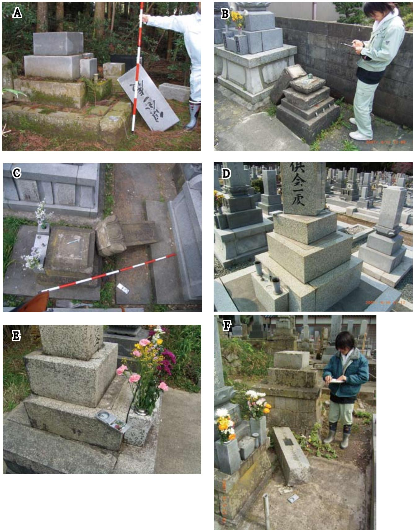
FIGURE 14. Field occurrences of displaced Wa-type and Obelisk-type gravestones. Directions of overturning of Wa-type and Obelisk-type gravestones are due to their horizontal sections as square. A-C, Overturning of Wa-type gravestones. D, Rotation of Wa-type gravestone. E, Translation of Wa-type gravestone. F, Overturning of Obelisk-type gravestone.
